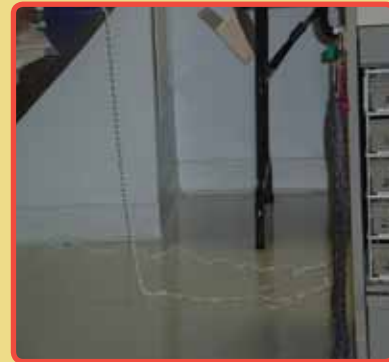
Figure 9.1. Loose phone cord
