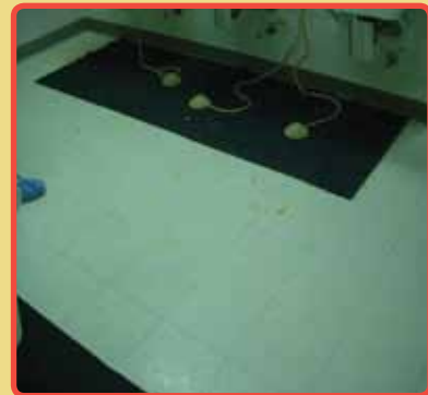
Figure 10.3. Mat is too small, contaminants present on the floor
