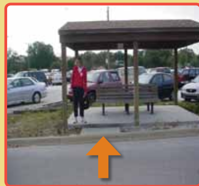
Figure 7.2. Uneven steps by shuttle bus stop, lacking a handrail
