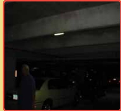
Figure 6.1. Dim lighting in parking area; light fixture is partially obscured by ceiling beams
