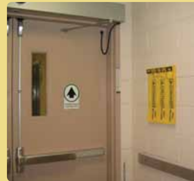
Figure 1.3b. Wall-mounted spill pads
